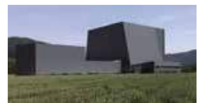
Pg. 111 Industrial plants. Oat processing plant
