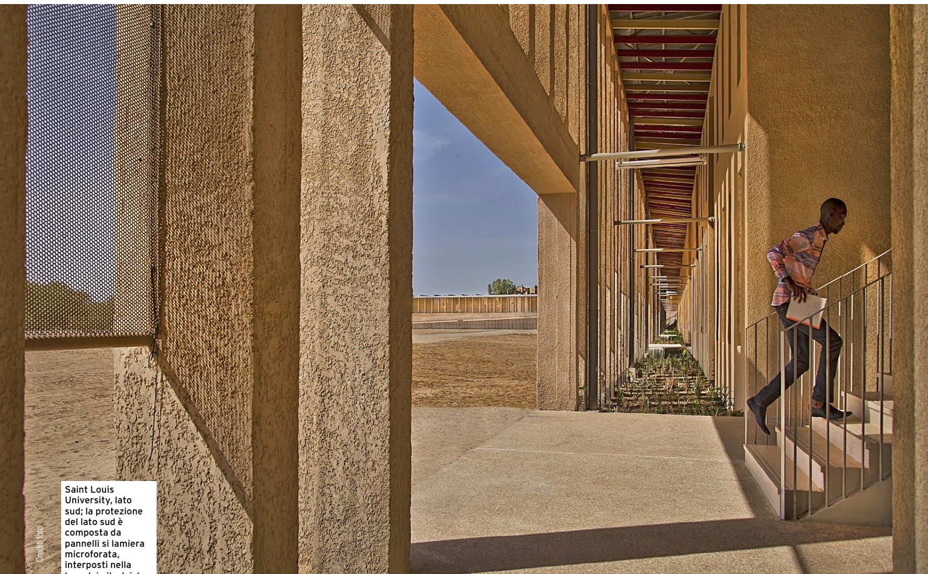
Saint Louis University: south side; the protection of the south side is composed of microperforated panels with the columns span. The distance, between the classrooms and the shield includes lemongrass plant
